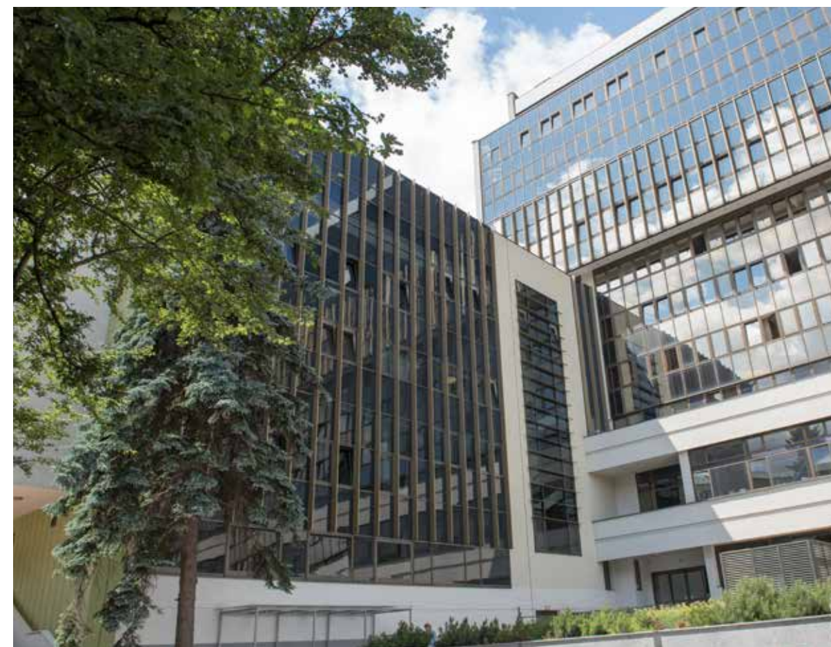
CTW – KNOWLEDGE TRANSFER CENTRE BUILDING (Al. Raławickie 14)
